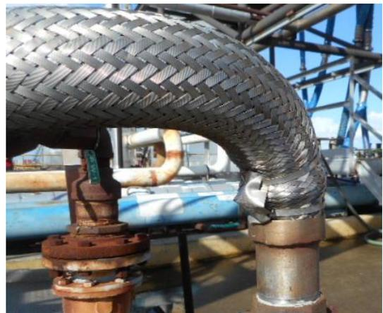
Clamps should never be put directly on the braided portion of the hose assembly. We recommend moving clamp to position past fitting attachment weld and onto pipe section, per the drawing below.
